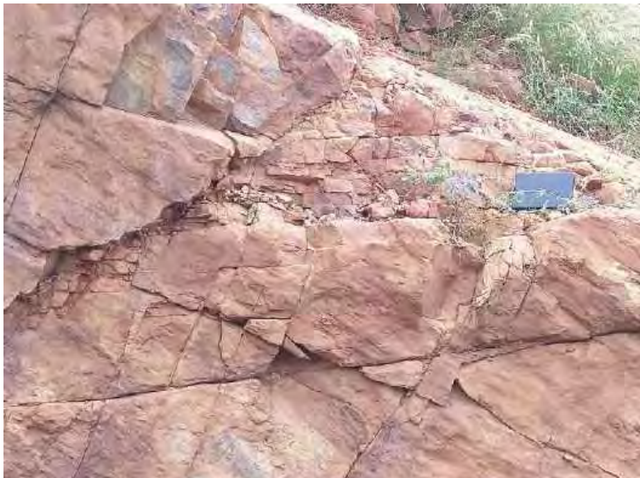
Figure 10: Multiple joint sets were observed throughout the area.
