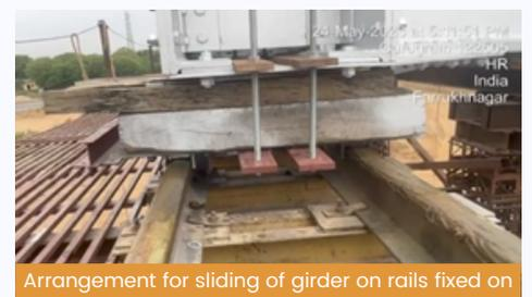
Arrangement for sliding of girder on rails fixed on launching girders.
